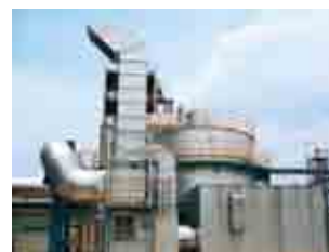
Regenerative thermal oxidizer installed at the Ichihara Works
