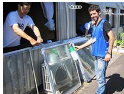
Applying film to outdoor double-sash windows
