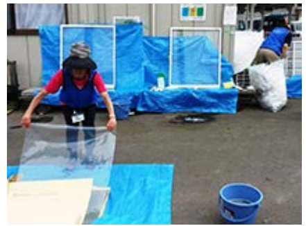
Each layer is sized to match and then applied to outdoor windows
