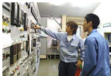
Intern being shown a control panel
