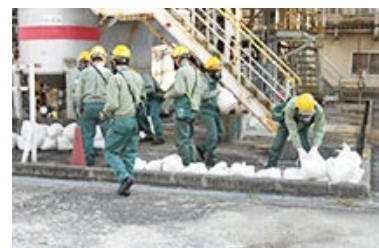
Stacking of sandbags to prevent leakage of material (Nagoya Works)
