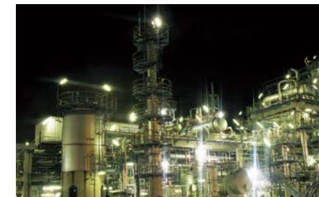
TAFMER™ manufacturing plant in Singapore
