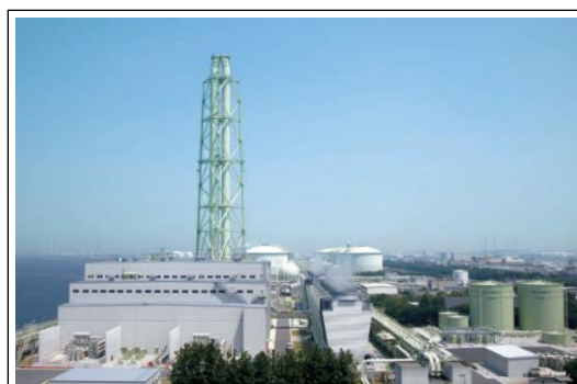
<Daigas Group's Senboku Natural Gas Power Plant>
