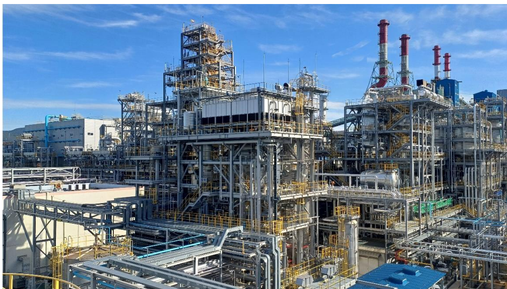
Kumho Mitsui Chemicals' Yeosu Plant
