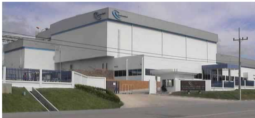
<Photo 2 : MHM's breathable film manufacturing facilities>
