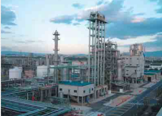
The new PP plant at the Osaka Works.
