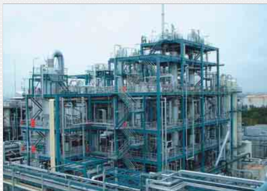
TDI Plant in Mitsui Takeda Chemicals' Kashima Works.
