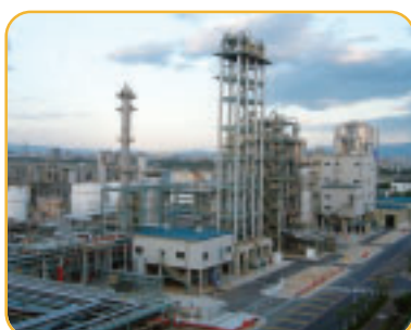
PP Plant in Osaka Works
