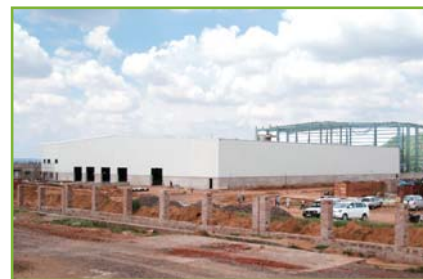
Production site under construction in India
