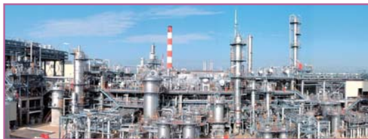
EPT plant with expanded capacity
