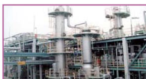
The new APEL™ production plant at the Osaka Works
