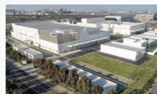
Newly completed plant in Taiwan
