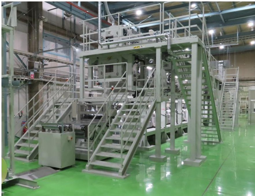
Demonstration facility for carbon fiber production
