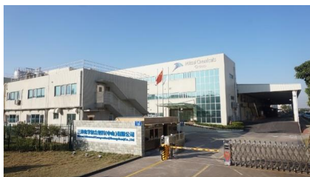
New facility site at Mitsui Advanced Composites (Zhongshan) Co., Ltd.
