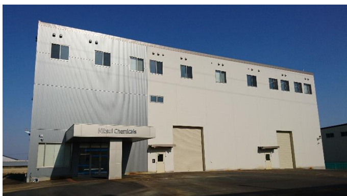
Exterior view of the Design & Solution Center
