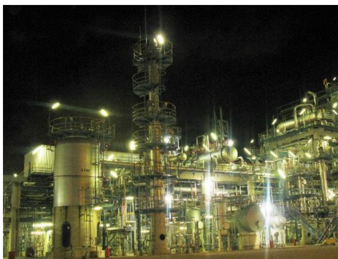
Singapore TAFMER™ Existing manufacturing plant
