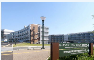
Research building of Kyushu University where MCI-CNRC is located
